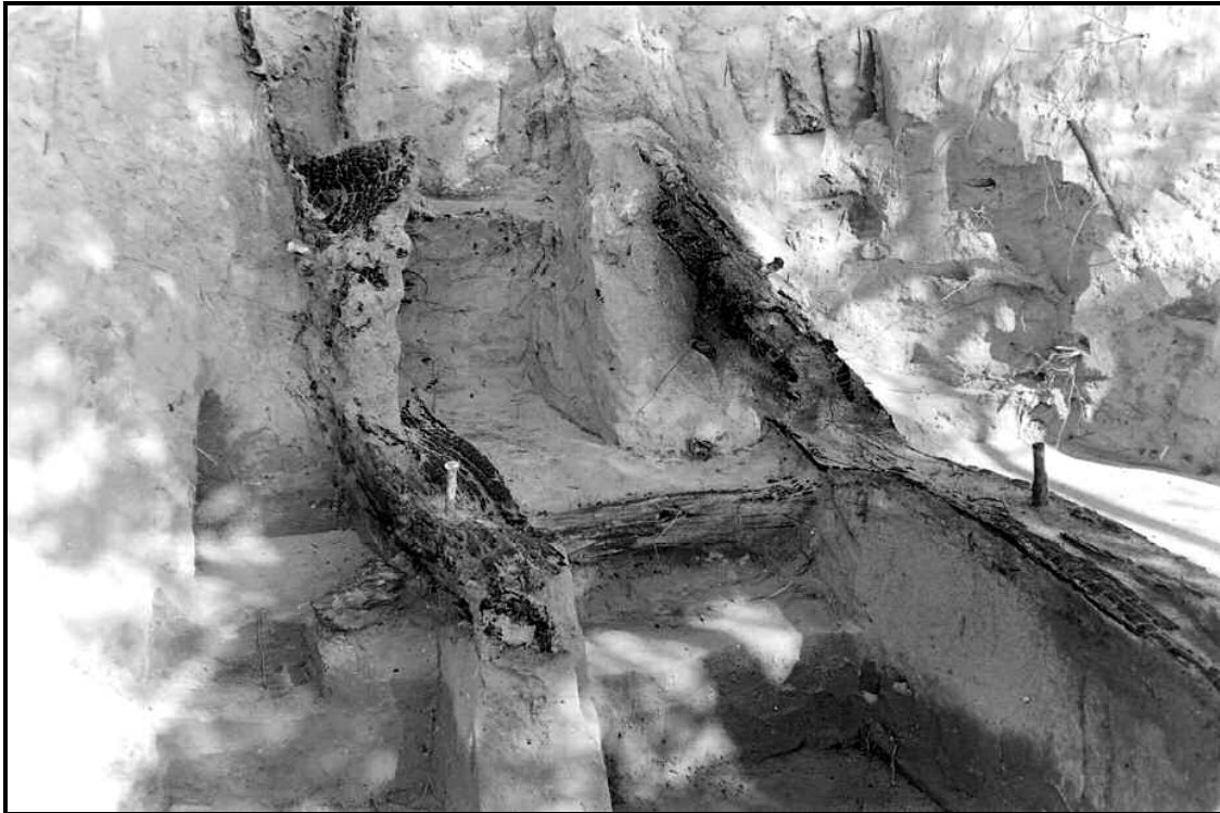
Figure 9: Sills along the entrance section of the bombproof were separated by two spacers dadoed to accept the sills.
