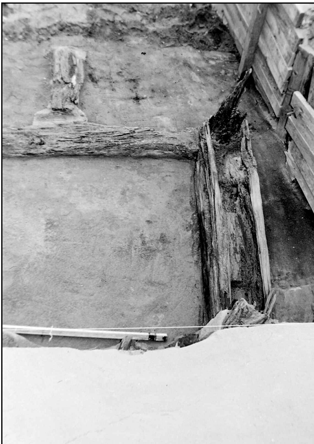
Figure 17: Mortices in the bombproof sills along the northwest wall were obvious once the studs were removed.
