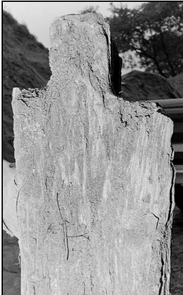
Figure 16: Tenons in the base of the 12-inch by 12-inch studs used in the bombproof wall were found to have been cut on only two sides.
