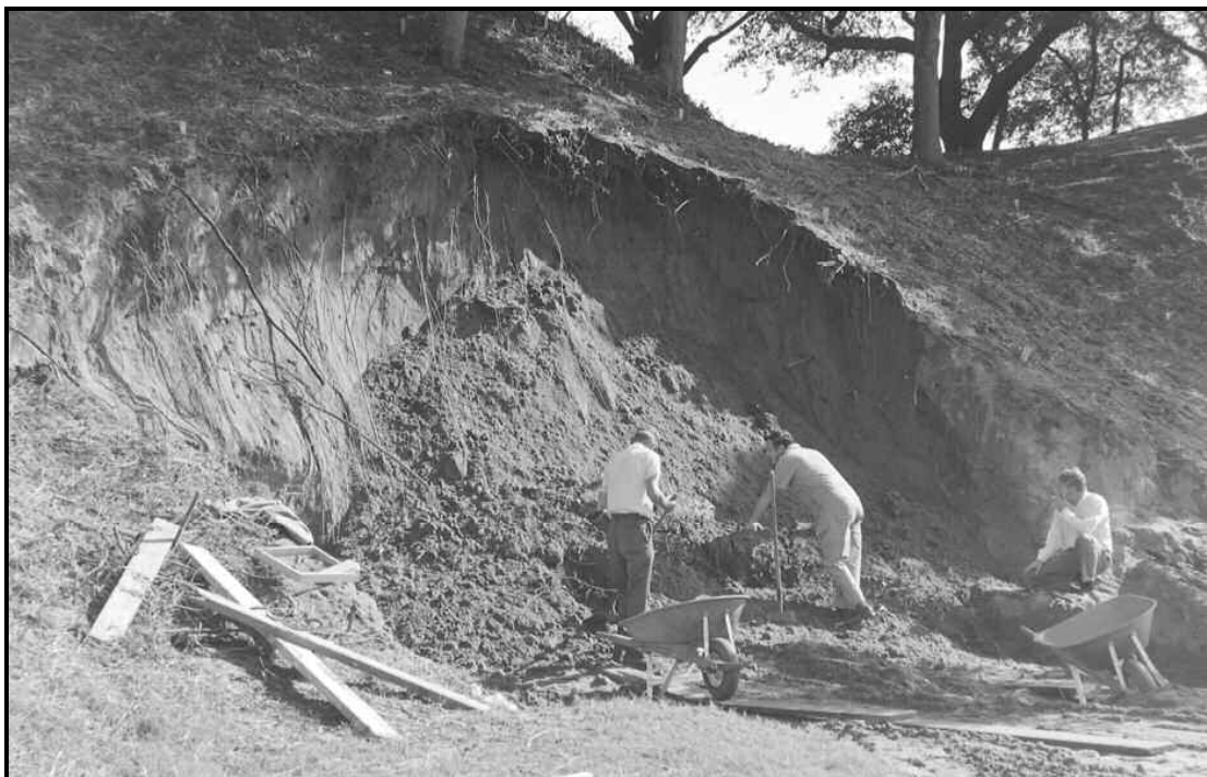
Figure 3: As the excavation proceeded into the traverse, cave-ins became more frequent and destructive.
