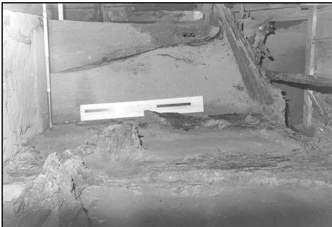
Figure 14: Excavation of the south corner of the bombproof revealed that the roof and walls had partially collapsed into the room once weakened by fire. A layer of charred wood can be seen directly above the original floor level.
