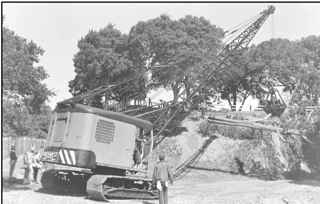
Figure 5: Final stages of excavation required the removal of several trees and approximately 500 cubic yards of overburden.
