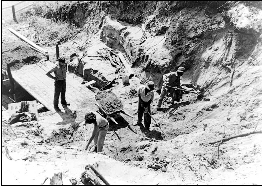
Figure 4: Prior to the availability of mechanical assistance, all overburden was removed by hand. A platform constructed over the bombproof entrance served both to protect the structure and facilitate loading a dump-body trailer designed by Fort Fisher State Historic Site.
