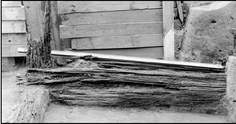
Figure 15: Corner posts were mortised into the overlapping timber of horizontal butt scarfs in the sills.
