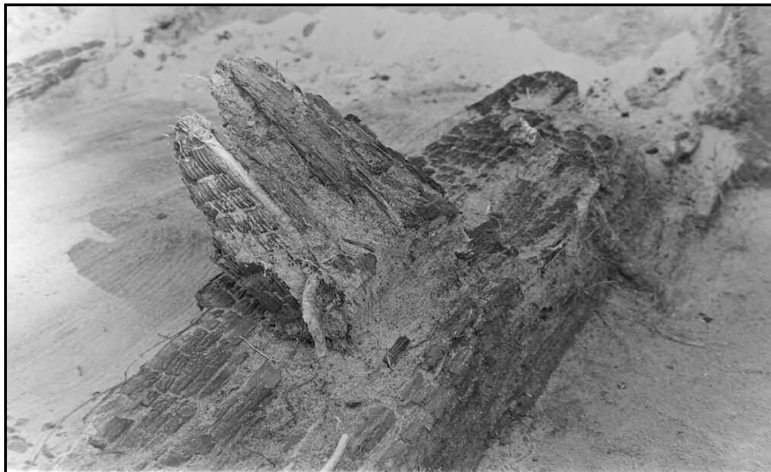
Figure 10: Wall studs along the entrance tunnel were found to have been set into the sills using stopped dado joints.
